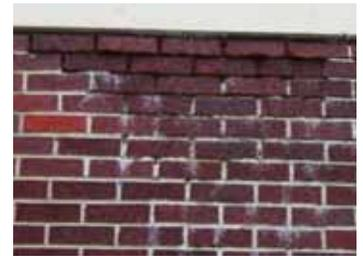
Brick deterioration from water
