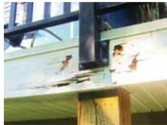
Wood rot from inadequate drip edge.
