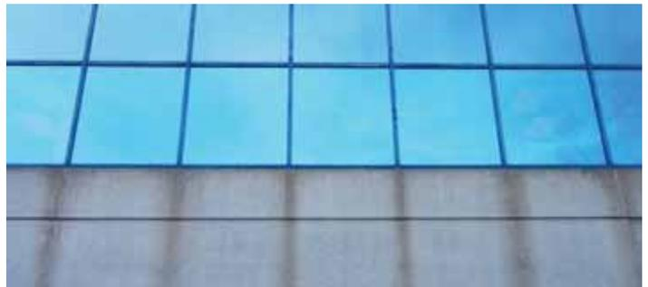
Water shedding can cause wall staining
