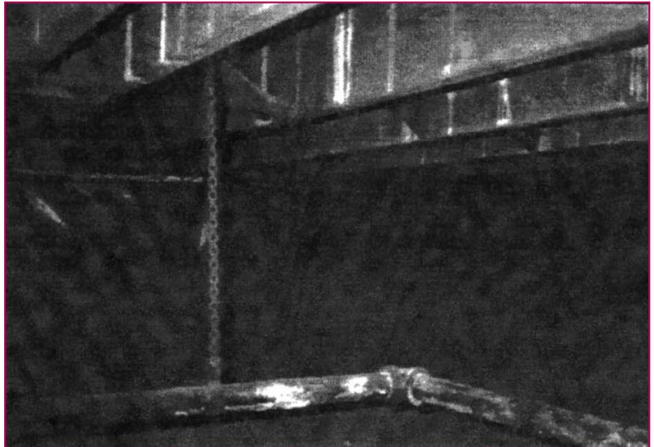
Crawl space post retrofit. New ground liner and ballast.
